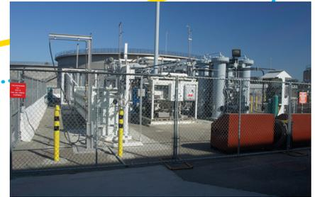
Air Products' Hydrogen Energy Station produces renewable electricity, hydrogen and heat from biogas.
